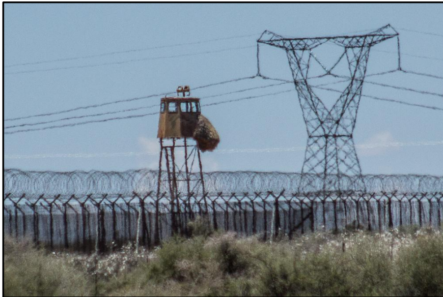
Fig 6 - Sociable Weaver colony on an abandoned lookout tower at Kronos Sub-station.
