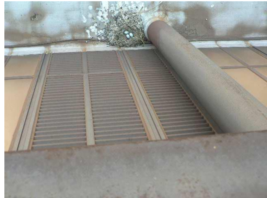
Fig 7 – Southern Bald Ibis nest on the ArcelorMittal building near Newcastle (Photo: Danie de Wet).
